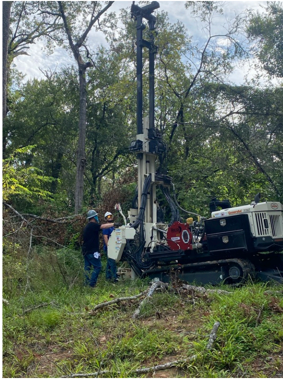
3. View northeast of SB-3 drilling activities
