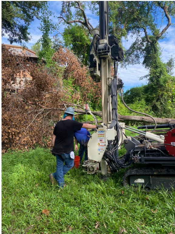
4. View west of SB-4 drilling activities
